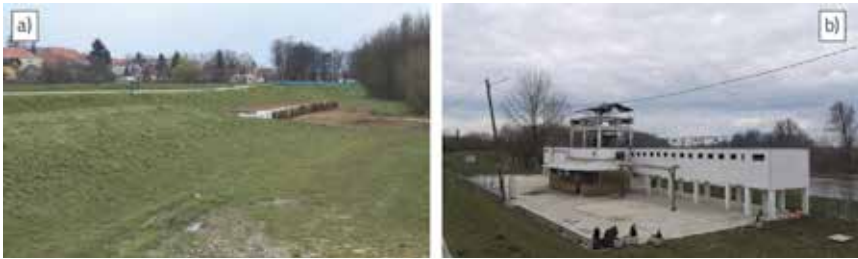
Figure 21. a) Subsidence of earth embankment at the approach to the bathing facility and (b) bathing facility in Petrinja along the Kupa River (b)
