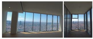
Figure 4. Photographs demonstrating insufficient number of operable windows on the façade
