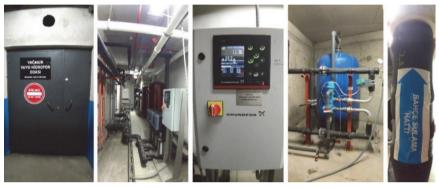
Figure 9. Building rainwater booster room and systems
