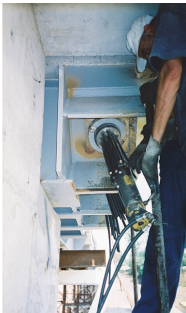
Figure 1 Cable tensioning by monostrand jack
